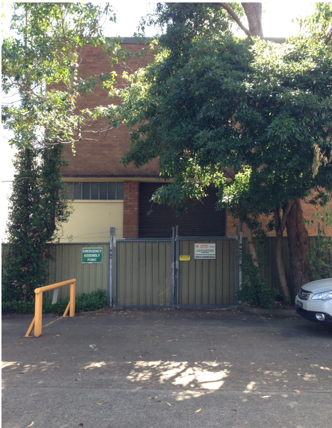
Figure 26 - View of Entry to Sydney Water building
