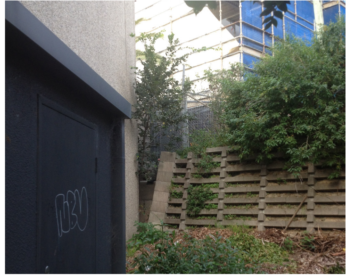
Figure 23 - Existing retaining wall
