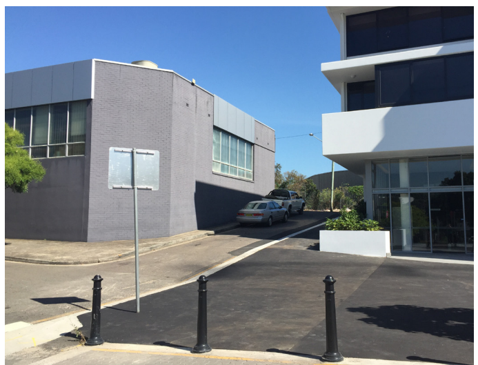
Figure 29 - Southern Entry to McPherson Lane from Merton St
