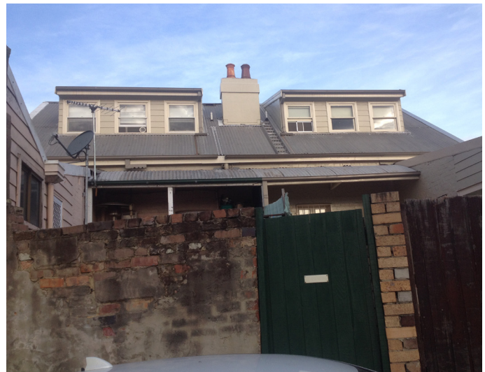
Figure 28 - Rear of heritage items from McPherson Lane
